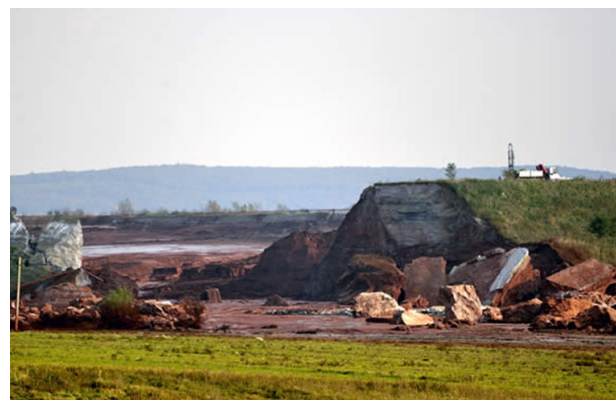
Image 2: Kolontar (Hungary). Failure of the ‘red mud’ dam retaining wall, 12 October, 2010. .
